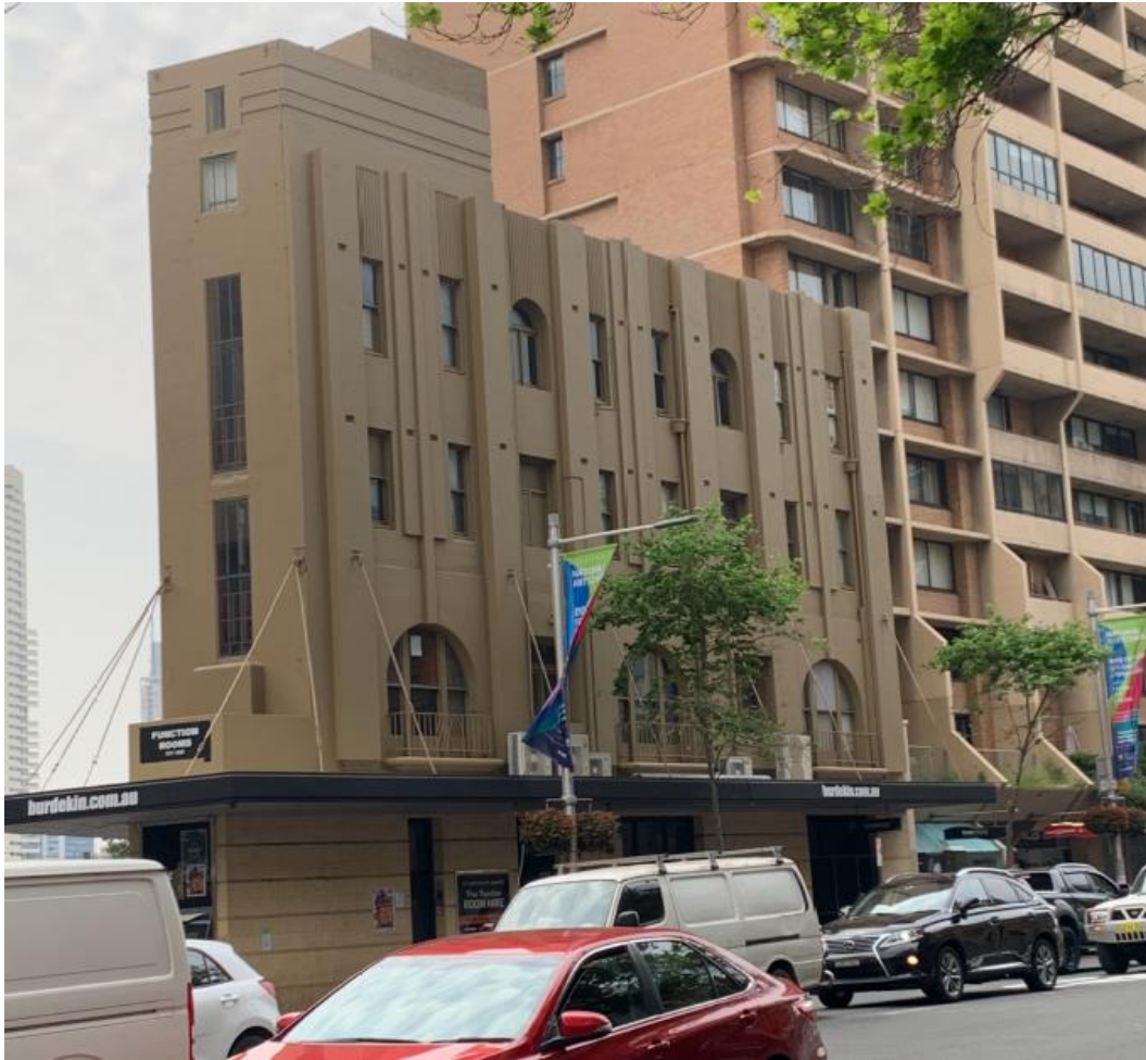
Figure 2: Site viewed from Oxford Street.
