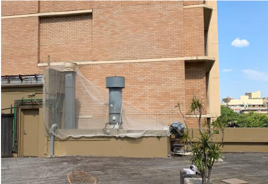
Figure 6: View from the subject rooftop facing east.
